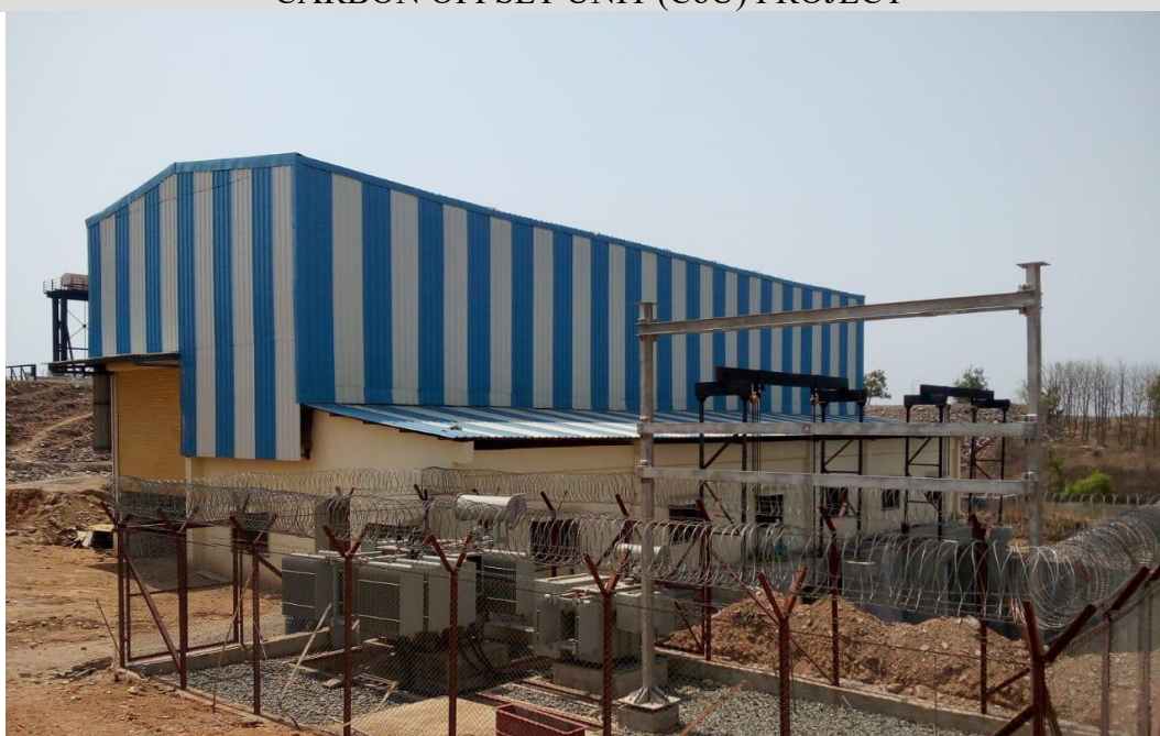
2.5 MW Gosikhurd Hydro Power Project
